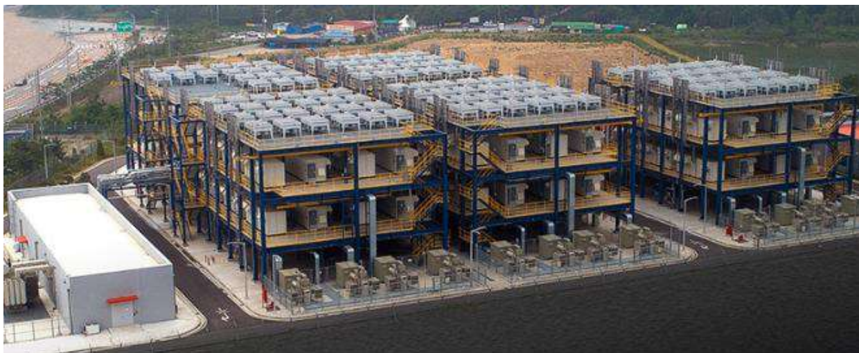
Figure 49: 50 MW byproduct-hydrogen-fuel-cell power plant located in Seosan, South Korea. [10]
