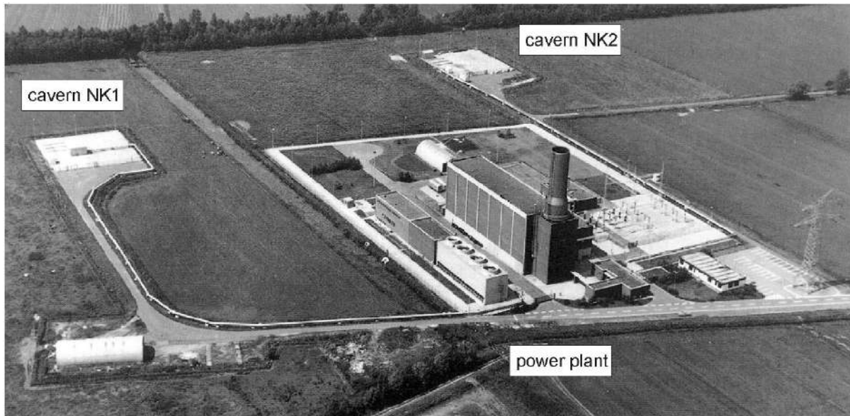
Figure 35: Aerial photo of the Huntorf facility [12].
