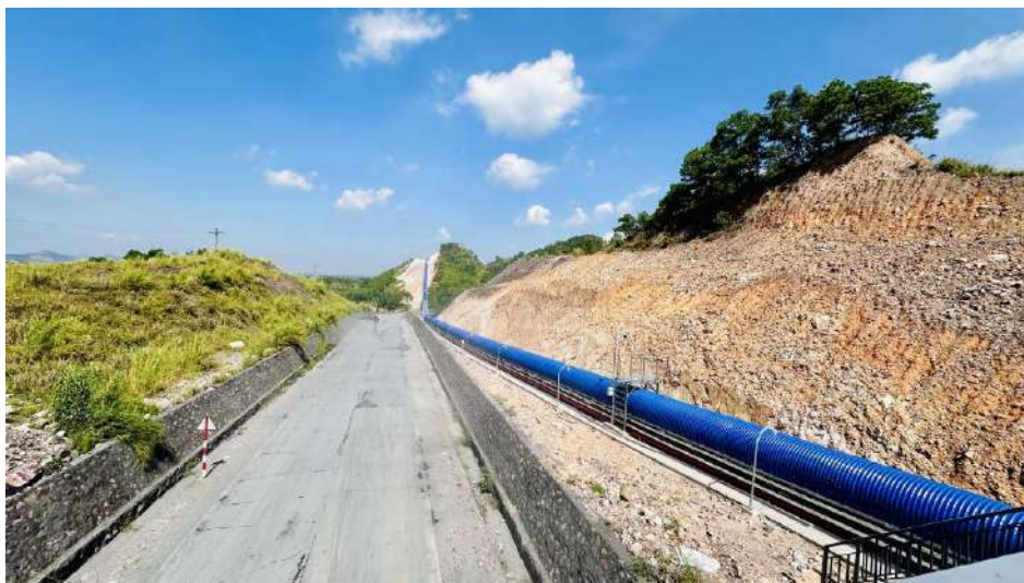
Figure 33: Trang Bach – Mao Khe coal conveyor route.
