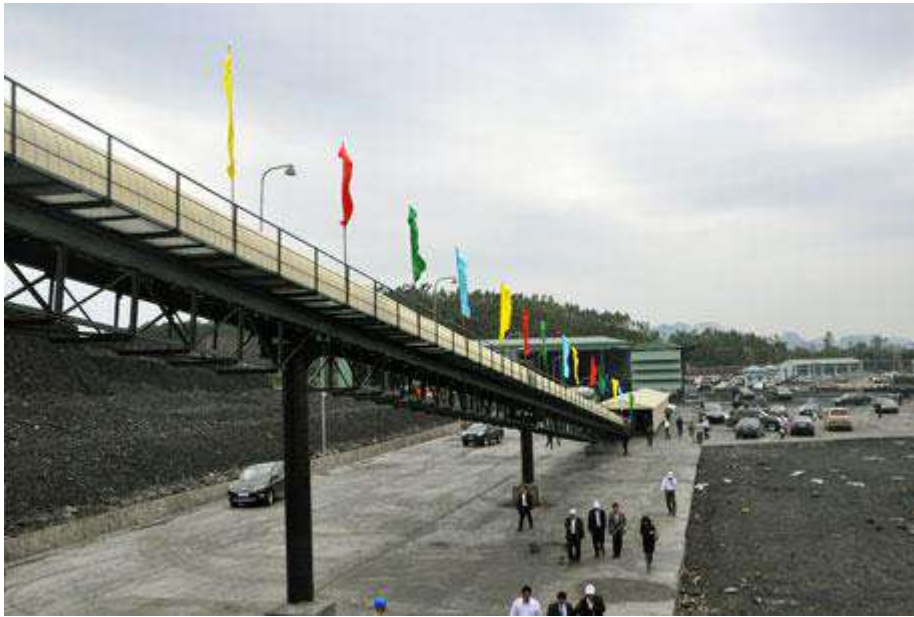
Figure 32: The coal conveyor supply system for Mao Khe Thermal Power Plant.
