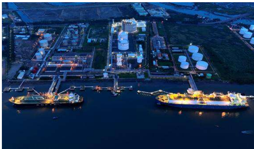
Figure 30: Image of Thi Vai LNG terminal
